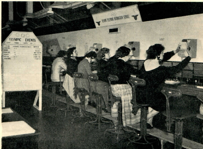
Fig. 17.—Telephone Information Bureau "MOLY 16".
