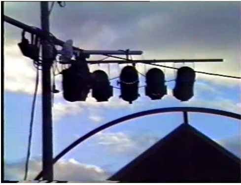
Photo : Penrith Mall Carols—FOH Lighting bars strapped to Streetlight poles
