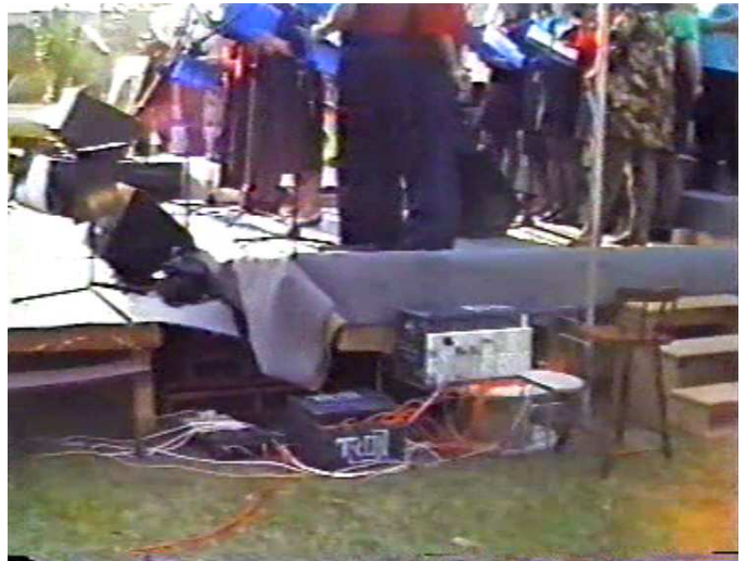
Photo : Emu Plains Carols. The PAMAC 12 channel dimmer rack and it’s associated 3 phase distribution board clearly seen, along with an empty cable drum which held the enormous length of TPS which formed the feed to the gig. Just to the right of the board is the earth stake—driven into the ground and bonded to the Neutral in an attempt to reduce “lazy neutral syndrome” on the long line.
