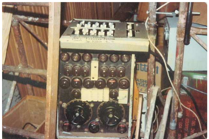
Photo from ACMS'80 showing one of Garth's massive Variac based dimmer panels built circa 1938. These were used for various specials and for house lights. As can be seen, each dimmer had three outputs, any of which could be switched to operate from the dimmer or direct from 240v – meaning that three separate channels in a rig could be dimmed using only one dimmer – and a lot of planning!
