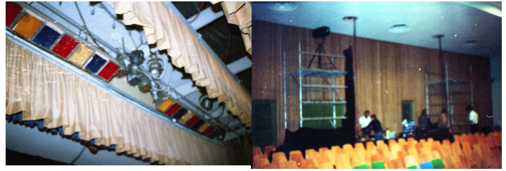
ACMS (Cooma) rig at Monaro High School circa 1982. The original Stand battens belong to the school's system and weren't used in the rig. The collection of Patt 123's and Patt23's were though. At the back of the hall.. Two scaffs for follow spots. Note the houselights removed to allow cables to be run through the roof. (Below) the luxury of a school hall with an accessible ceiling space. The heavens in heaven!
